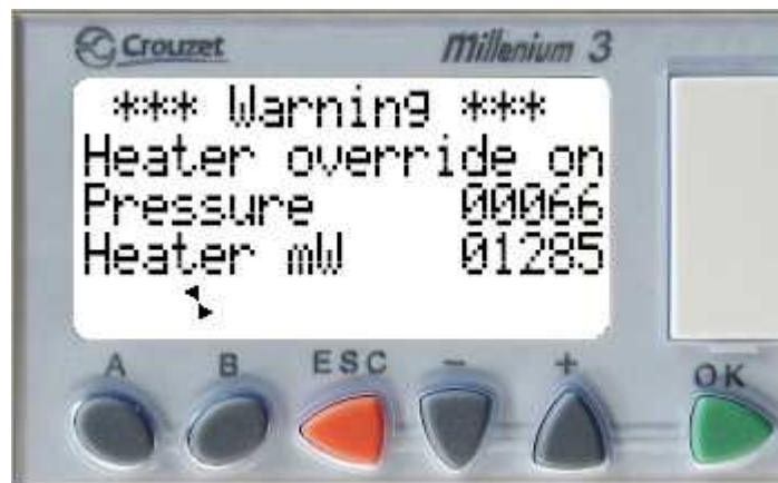
Fig 6-5 Screen display if the PT2 heater is fully energised
