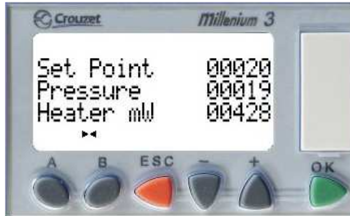
Fig 6-1 Power-on display which is also the default operational display, termed "normal" mode
